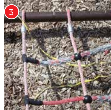
3 Worn ropes and an exposed anchoring device make this component unsafe.
